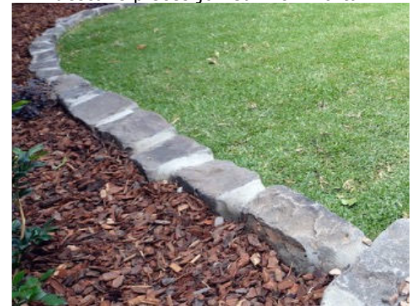
Bluestone pieces joined with mortar
