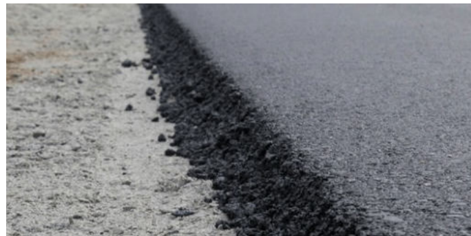
Compacted crushed rock with a curved mound 200mm
